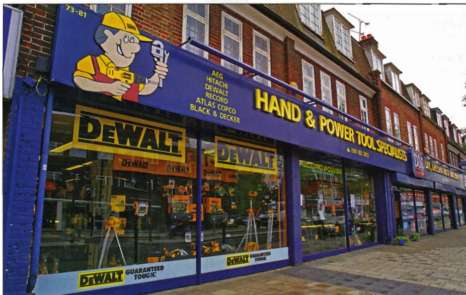
▲ D&M Tool Store began as a double-fronted shop, but expanded to take up five buildings
