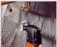
Ideal for dismantling installations that are no longer required. Using the universal E-CUT saw blades the pipes are clipped off for subsequent grouting flush to the wall.
